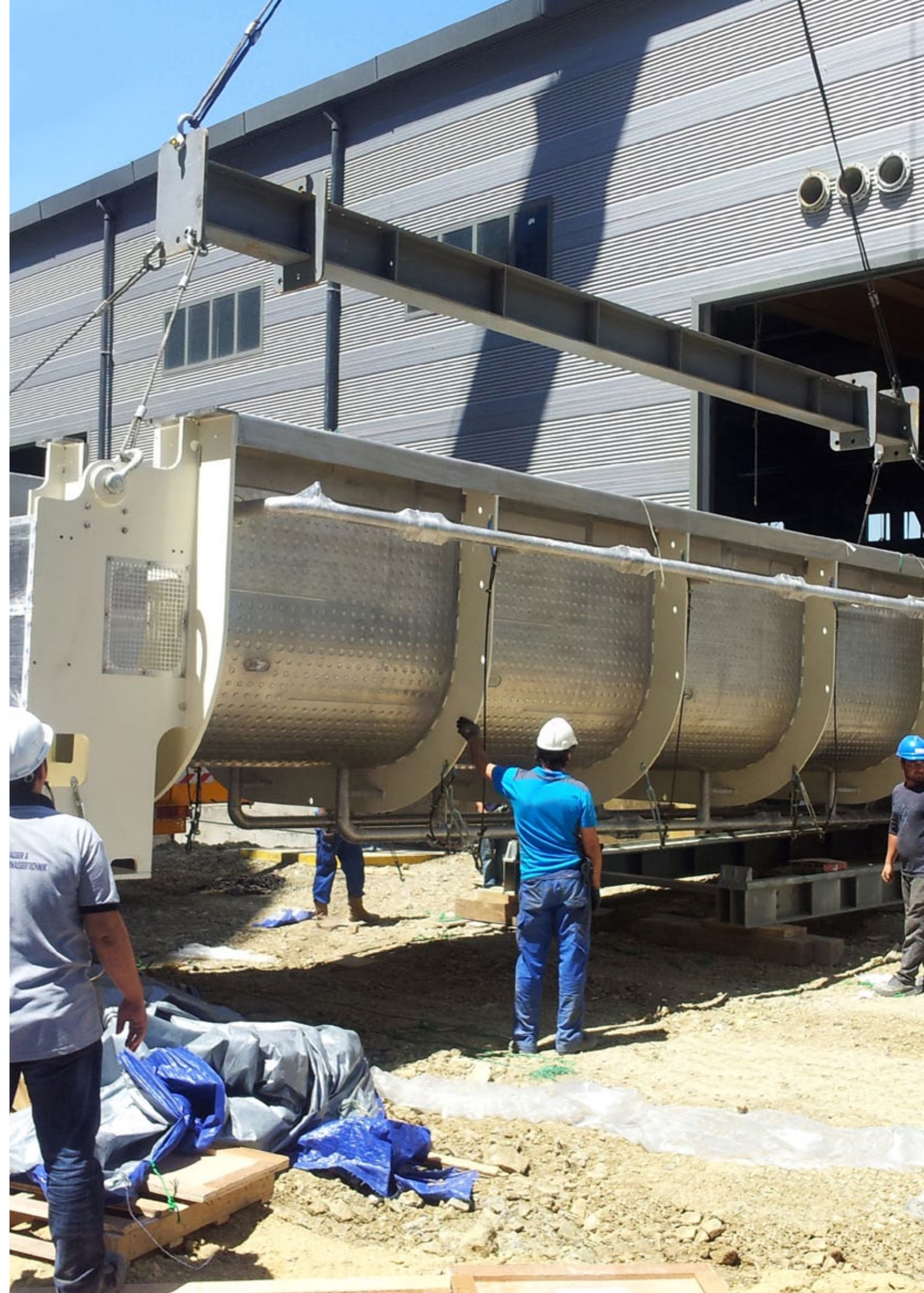
Installing a paddle dryer ▶
