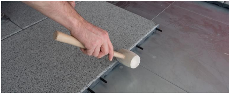
Closing the gaps with a hammer
