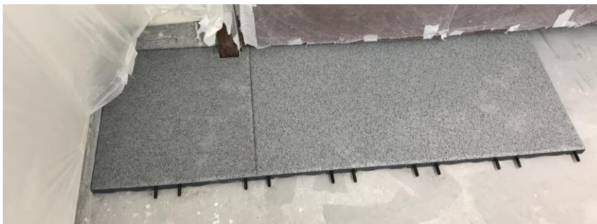
Installation of the tiles along a wall with the connector pins towards the next row
