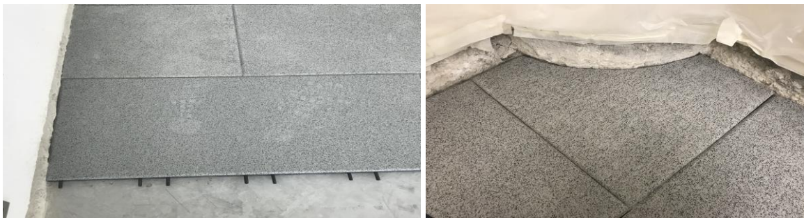
Each row should be offset by a half tile; tiles can also be cut around curves
