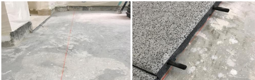
Creating chalk lines and laying the tiles along this line
